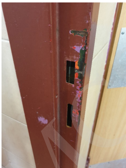
Figure 5. Peeling paint in the boys' bathroom – a photo taken by an activist and submitted as part of the retrial
